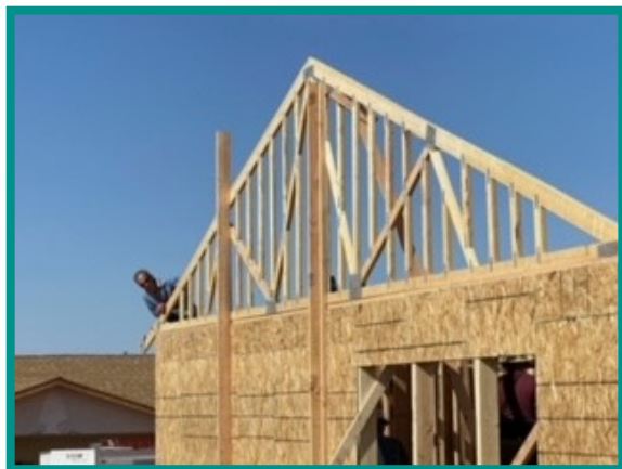
First roof truss going up
